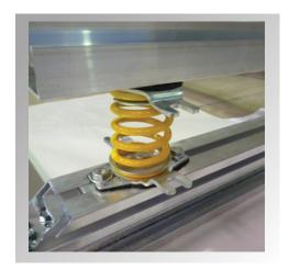
Fan and motor assemblies are mounted on a common extruded aluminium base located inside the air handling casing which in turn is mounted on anti vibration mounts designed for 93% isolation.
