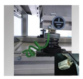
Fan motor assembly isolated by anti-vibrators and flexible connectors shall be earthed to the casing. Further, the casing is earthed as a part of field wiring to ensure complete safety. Fan section access doors shall be incorporated with safety "cut-off" switches electrically interlocked with the fan motor. No sharp edges, all projected screws shall be covered with nylon caps.
