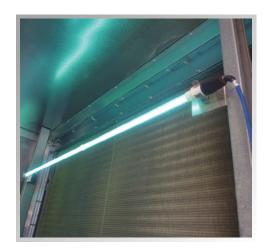
Ultra Violet lamps use Quartz (lamps)and are filled with Mercury vapour. UV lamps improve energy savings and reduce maintenance by keeping the coil clean. UV lamps can be installed either upstream or downstream of the cooling coil. UV lamps are also available with reflectors for better efficiency.
